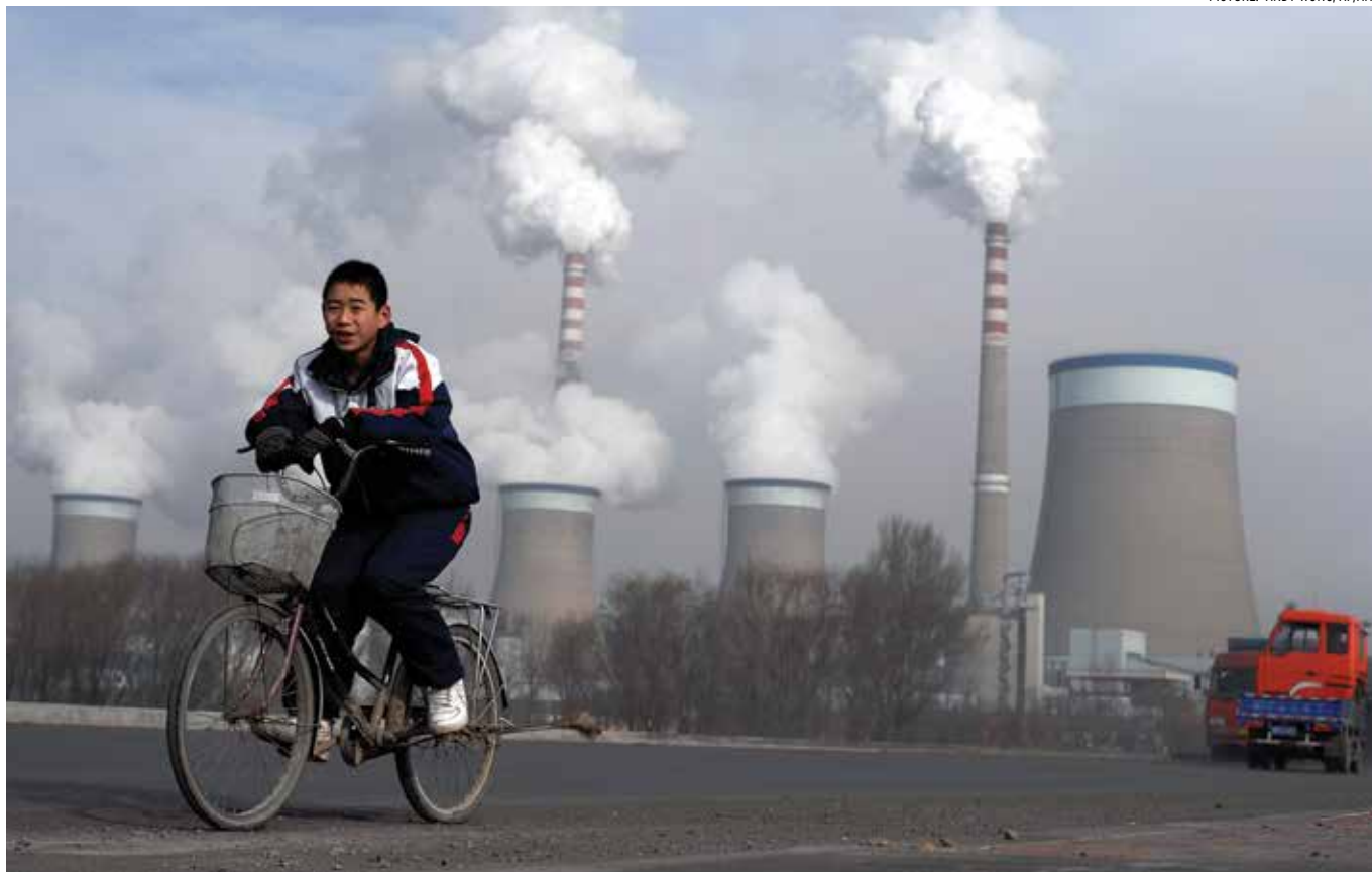
A Chinese boy cycles past the cooling towers of a coal-fired power plant in Dadong, Shanxi Province, in 2009. Coal has been the principle fuel of China's spectacular economic growth in recent decades but will need to be toned down if China is to curb its emissions intensity.
