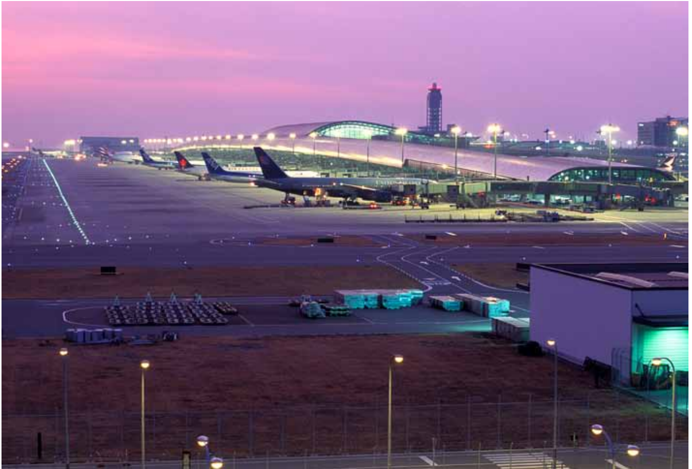
Kansai International Airport, one of three specifically targeted for privatisation under legislation passed in 2013. One potential benefit is the introduction of unified management to airport operations, in contrast to the accepted practice whereby buildings, car parks and the airport apron are run by different bodies.
